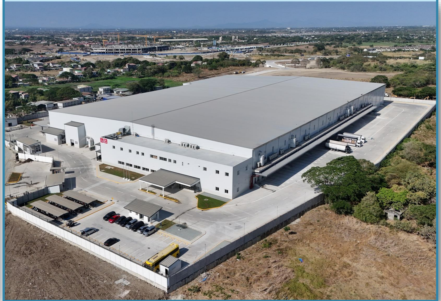
Uniqlo Logistics Facility in Riverpark, General Trias
